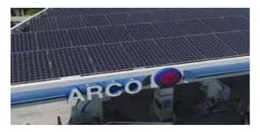
Additionally, the shade structures and canopies over the fuel pumps are ideally suited to accommodate the solar panel arrays; solving a major challenge otherwise presented by the relatively large real-estate space needed to host these solar system panels.
